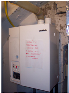
Small boiler (caldaietta) and the indicative perimeter of warmed area
