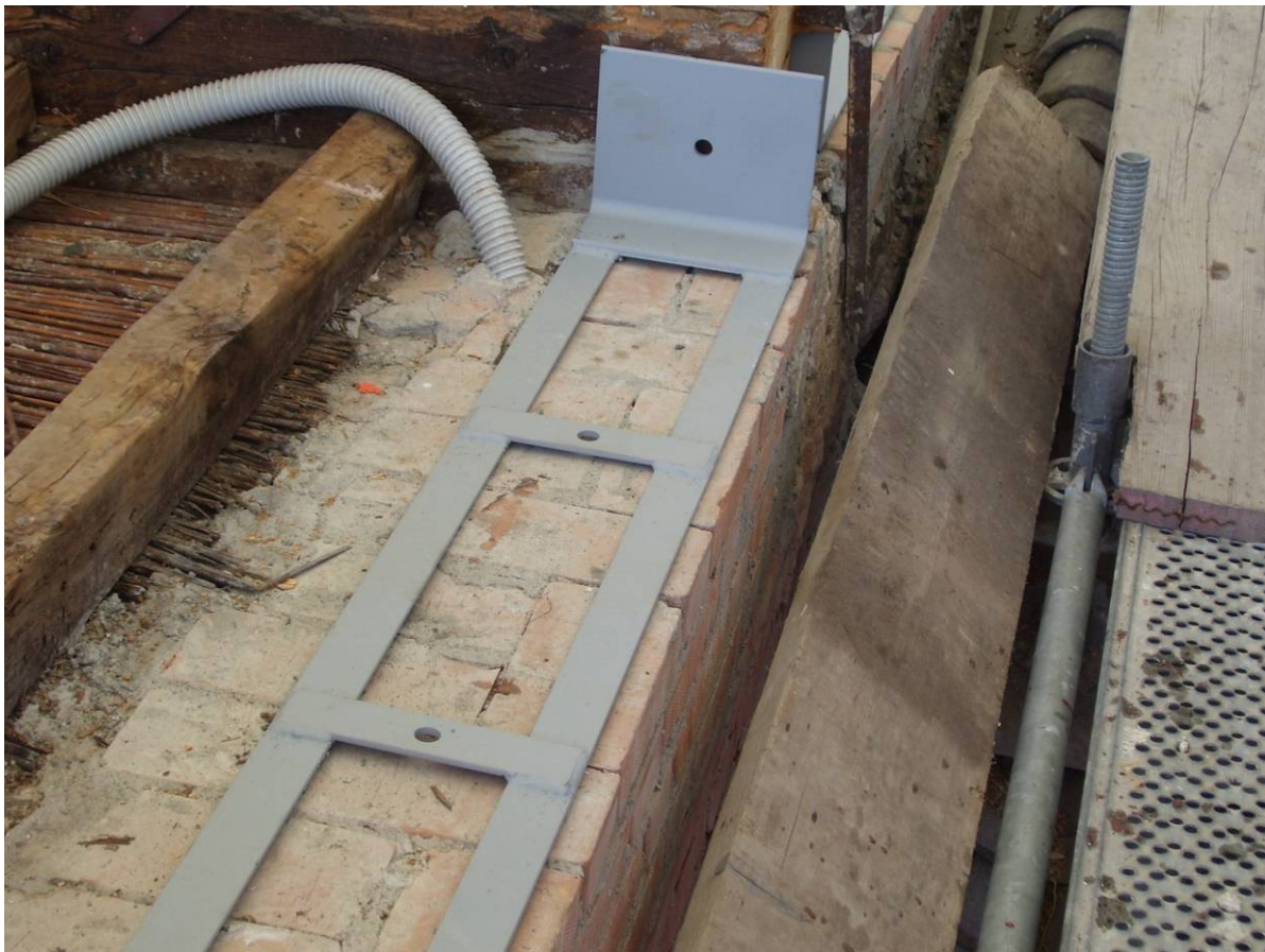
Fig. 41-42: metal curb for the consolidation of perimeter walls
