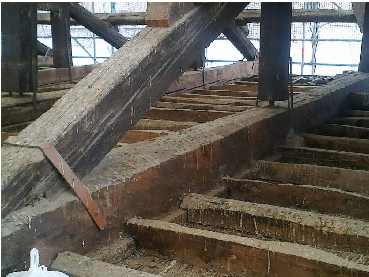
Figure 35-36: Deterioration of the wooden structure of the roof
