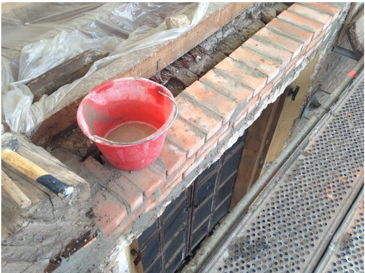
Figure 37-38: ancient chimneys and intervention of consolidation of the masonry
