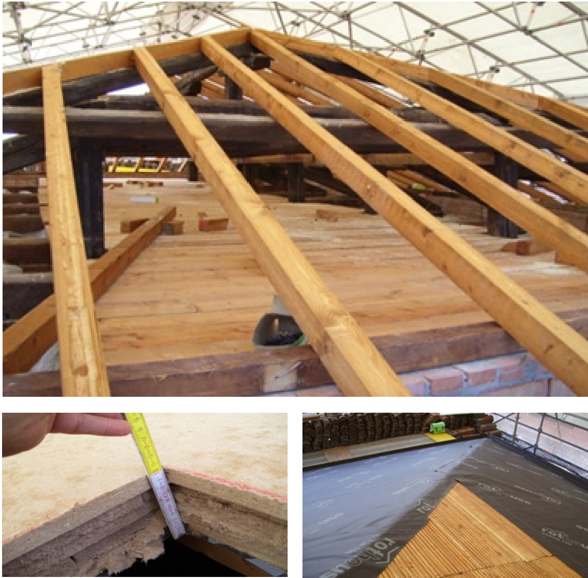
Fig. 43-44: replacement of the wooden beams and installation of insulation on the roof
