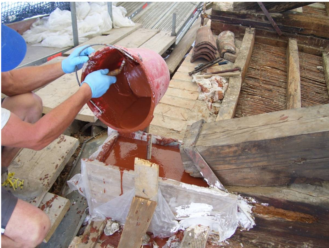
Fig. 39-40: wooden truss gear and consolidation with steel bars and resins
