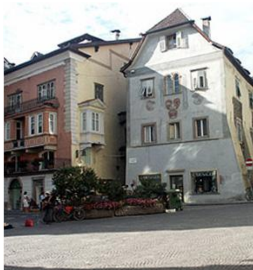
Picture 3.3: Weighhouse, Bolzano, Italy
