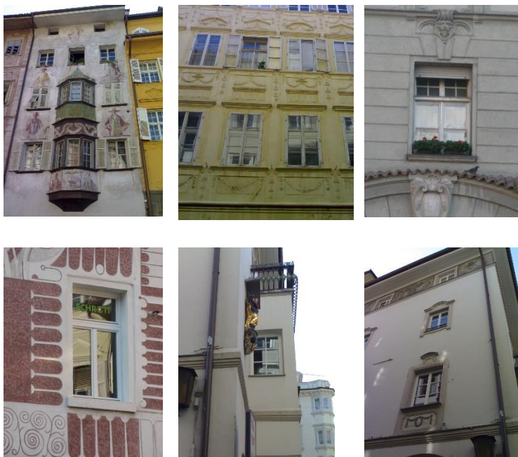
Figure 1-6: Originally, the wooden frames, impost and sash bars were very fragile and thin, possibly moulded (fig.1-3), while the optic of the typical replacements is much broader (simple application of the IV68 standard, fig.4-6).
