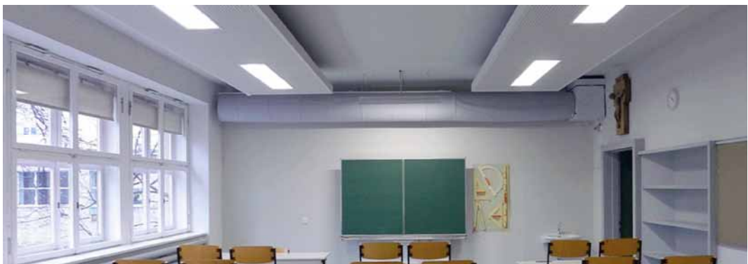
Figure 13. Active overflow ventilation in prototype class room in Innsbruck (A), textile diffuser and fan.
