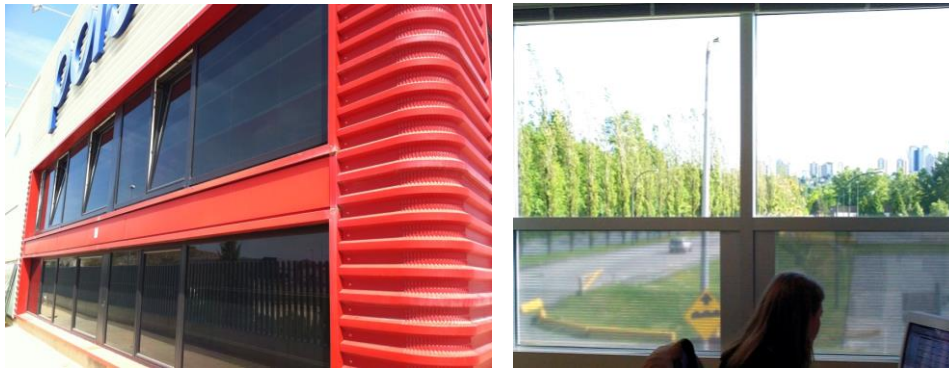
Figure 9: Double-glazed PV glass with filter properties for solar control and acoustic isolation.
