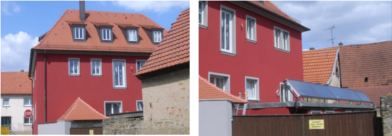
Figure 6: Kleinlangheim, Bavaria/Germany (Hans-Christof Haas, BLfD), The solar panels is almost not visible from the street. It was not installed at the main building but on an annex.
