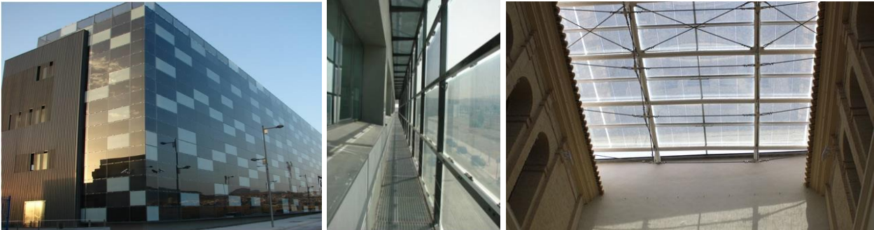
Figure 4: Left and center: Double skin with semitransparent PV glasses with security profile. Right: Atrium.
