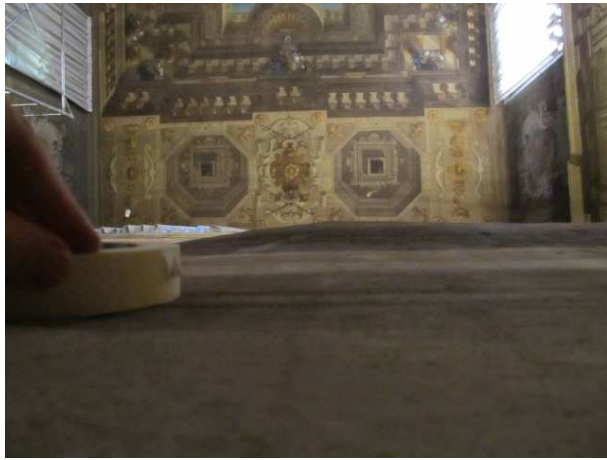
Figure 1: Documentation of room envelope, here: walls are not completely flat (view to the ceiling)
