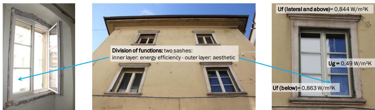
Figure 2 At the “smartwin historic” prototype, installed at the Public Weigh House in Bolzano, the two functions “energy efficiency” and “aesthetics” are realised in separate layers
