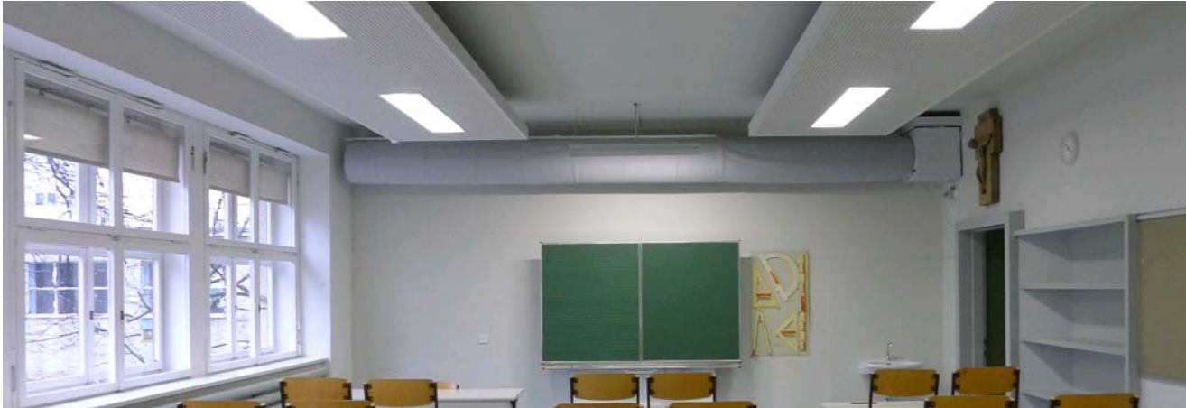
Fig. 2: Silencer and fan-box prototype manufactured by ATREA
