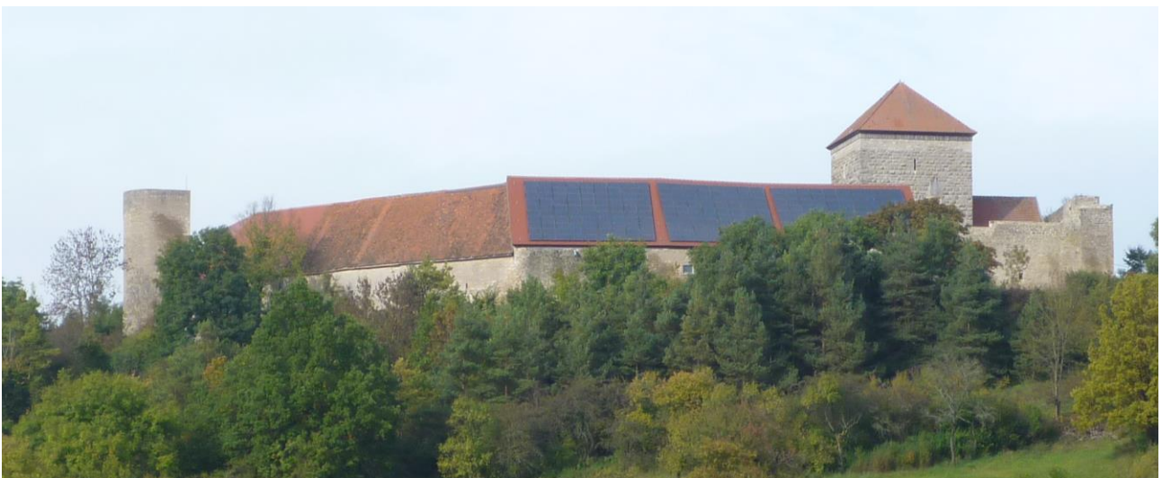
Figure 4: Castle Brauneck, Baden-Württemberg/Germany (Hans-Christof Haas, BLfD). The homogeneity of the roof is lost by installation of the PV system. Furthermore the castle has with its exposed position a high long-distance effect.
