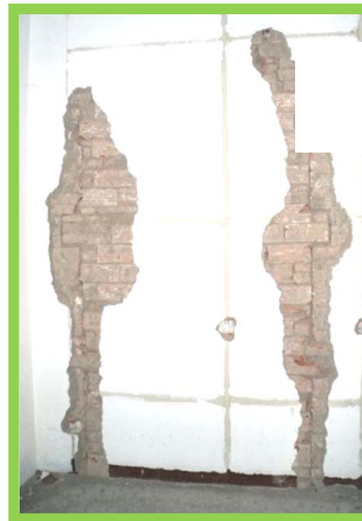
Identification of chimney flue
