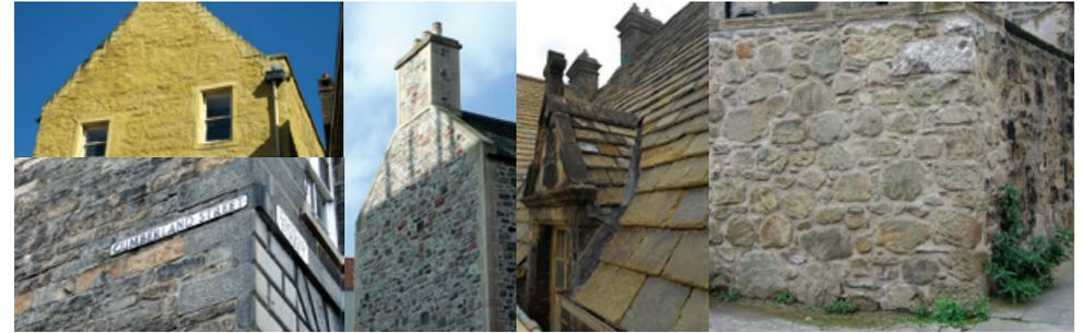
*The sense of place in the World Heritage Site is strengthened by the quality, durability and consistent use of local materials for construction, including local sandstone, Scottish slate, lime plaster, cast iron, timber and glass.*
