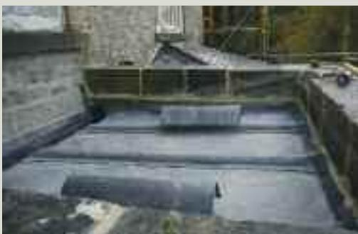
*A recently re-covered lead flat roof. These modern lead roof vents were introduced as, previously, poor ventilation had caused moisture to build up within the roof space leading to timber decay*
