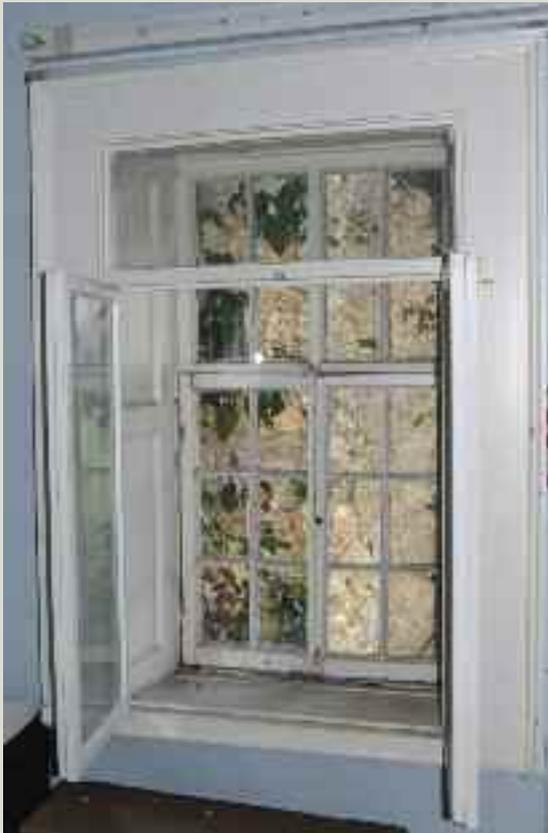
*An Edwardian window with 1950s secondary glazing. The secondary glazing is chunky and does not match the original window profile and blocks light from the room. The position of the frame within the opening prevents the shutters from being used*
