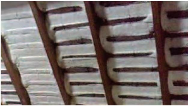
**72** The use of sprayed foam to avoid a 'nail-sick roof' and provide some insulation is not recommended good practice on a historic building
