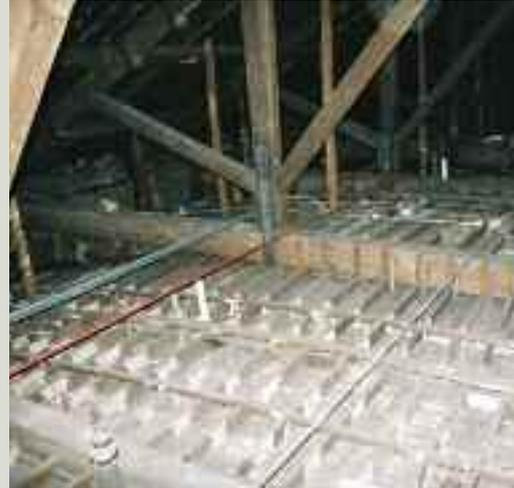
*A large roof space with no insulation above the ceiling; while the heat rising from the building interior may benefit the timber and other building materials in the roof space, a lot of energy is wasted in this way*
