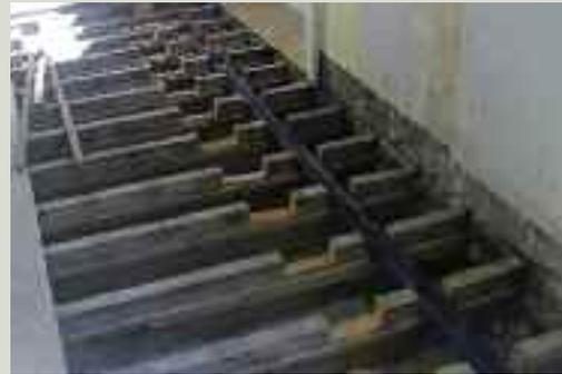
*Existing holes in floors or notches in joists can be reused to accommodate new runs of services. New holes or notches should not be created to avoid further weakening of the joists which has occurred in this example. Where there is existing pugging within the floor space, it should preferably be left in place*
