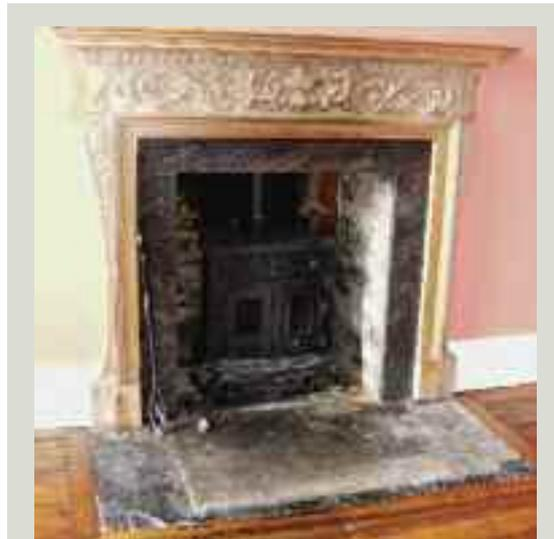
*Wood-burning stoves can be efficient but in a traditional building they should generally only be fitted into non-decorative fireplaces. Historic grates and fire surrounds should not be damaged or removed in order to fit a stove*
