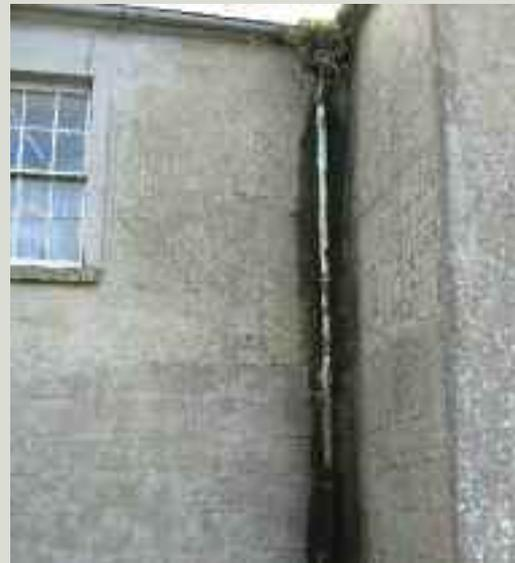
*The importance of maintaining rainwater goods in good working order cannot be over-emphasised. Not only will the water running down this wall cause rotting of the building fabric and damage to the interior in the short to medium term; the dampness in the wall will also cause it to transmit heat more quickly from the inside of the building making it colder and less thermally efficient*
