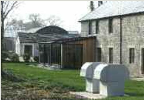
*Air-to-water heat exchangers: a heating system provided to a converted stable building. The grey metal casing will be camouflaged by future planting*
