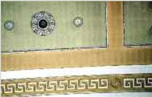
*This plastered ceiling has no insulation above it. Discolouration can be seen on the plasterwork between the timber joists located above, as the timber is slower to transfer heat to the cold roof space than the plaster alone. Dust particles in the warm air passing through the plaster remain trapped on the surface causing the discolouration*
