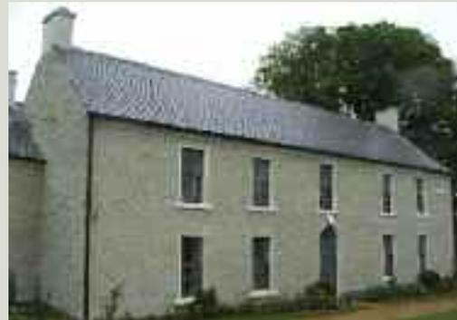
*A lime-rendered façade, in good condition, improves the insulating value of a wall and prevents damp penetration to the inside of the building*
