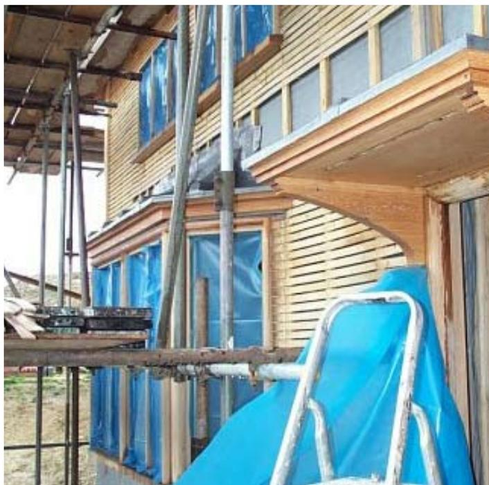
Front elevation of the newly insulated timber frame prior to rendering
