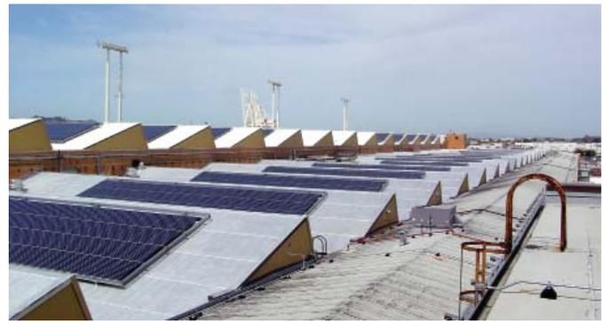
Fig. 23. Solar collectors installed in a compatible manner on low sloping sawtooth monitors. Top Photo: Neil Mishalov, Berkeley, CA.
