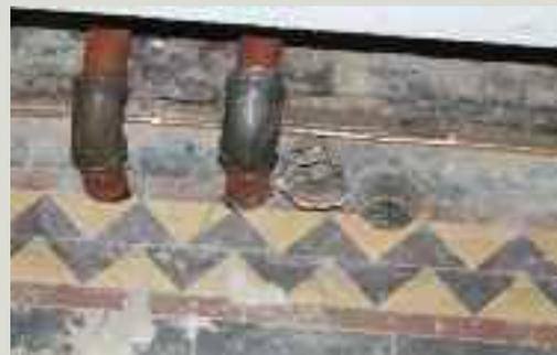
*New and redundant holes in floors should be made good, fire-sealed where appropriate, and finished to match the existing floor. Where new service runs would interfere with the fabric of a protected structure, planning permission may be required*
