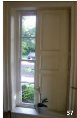
**52** Air infiltration through a sash window in good condition can be reduced by as much as 86% by adding draught-proofing
