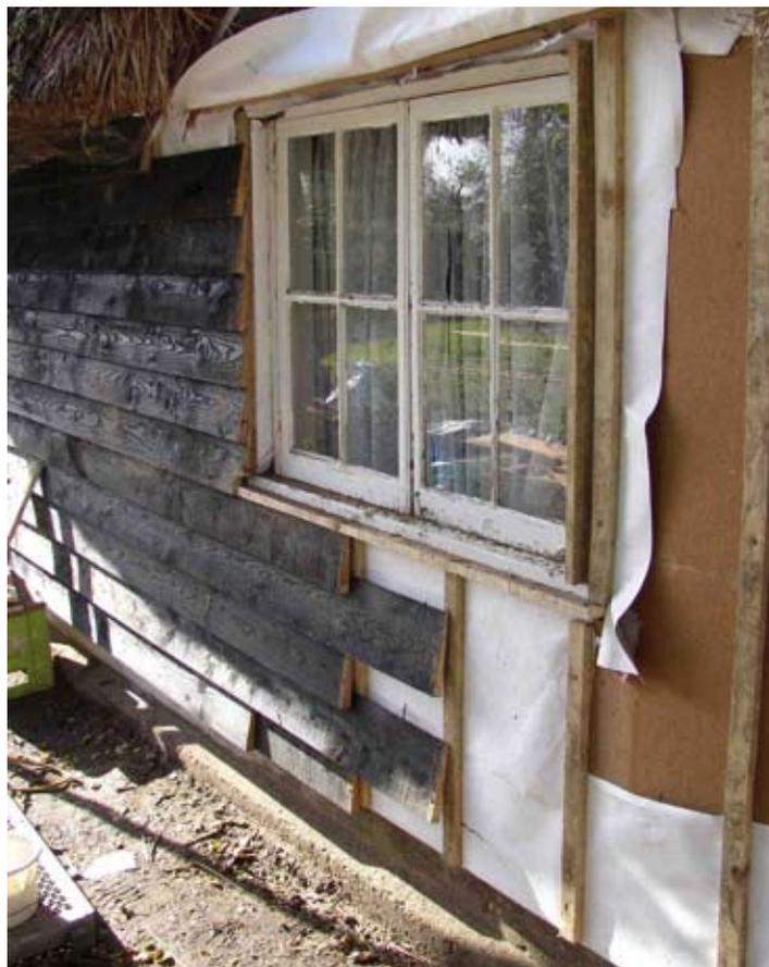
Rear elevation showing works: The woodfibre board can be seen behind the weatherboarding. Junctions are dressed with vapour permeable roofing felt to reduce the risks of draughts
