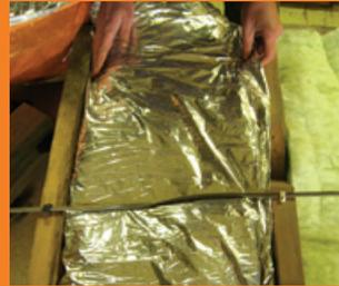
It is very important to draught-proof and insulate your loft hatch as well in order to have a continuous insulation without gaps. Insulation must also go over the water tank. Cables should run above the insulation (on the cold side) to avoid overheating. Also remember to add lagging around pipework to avoid frozen/burst pipes.
