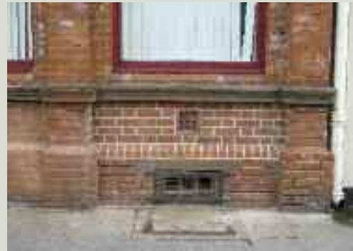
*A floor vent to ventilate the ground floor was built into the wall between the cellar and ground floor windows as part of the original design*
