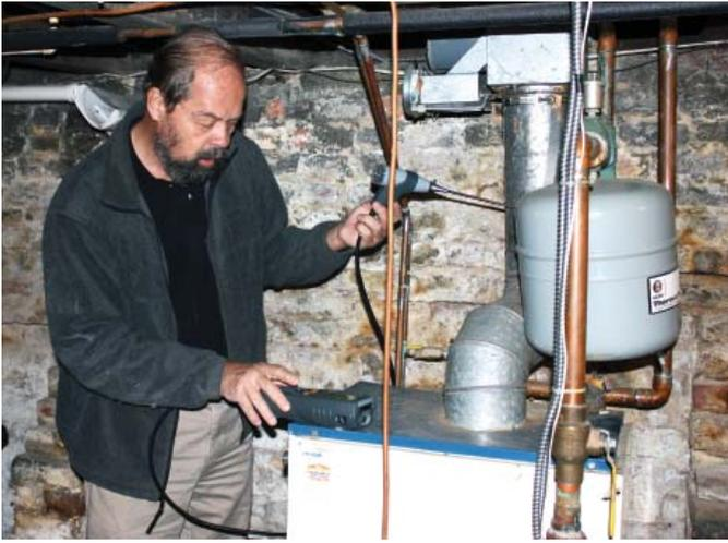
Fig. 9. An energy auditor tests the efficiency of a boiler.
