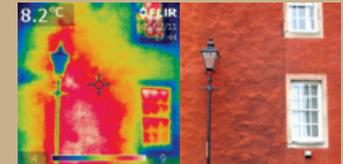
The defect in the insulation allows heat and dampness to escape through the fabric, damaging the wall.
