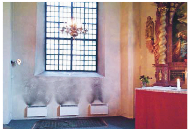
Figure Soiling in the vicinity of a radiator in a church.
