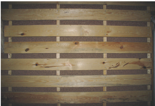
Figure 9 interior insulation System (insulation loam cork) Warehouse city in Potsdam.
