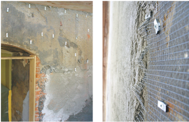
Figure 6a, b Safeguarding baroque plaster under heat insulation plaster
