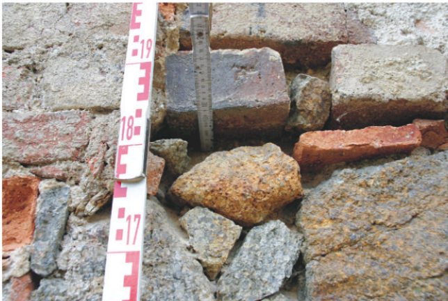
Figure 5 Heterogeneous masonry, missing joints
