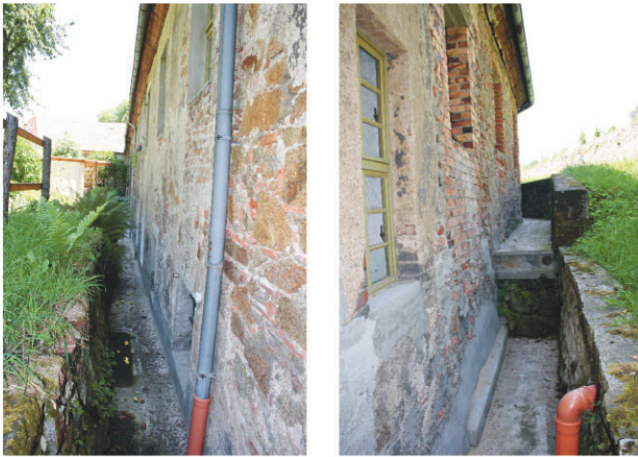
Figure 4a, b A trench at the north facade functions as interspace to the soil.
