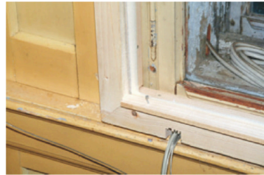
Figure 5 Window situation in the ground level equipped with a third window level.
