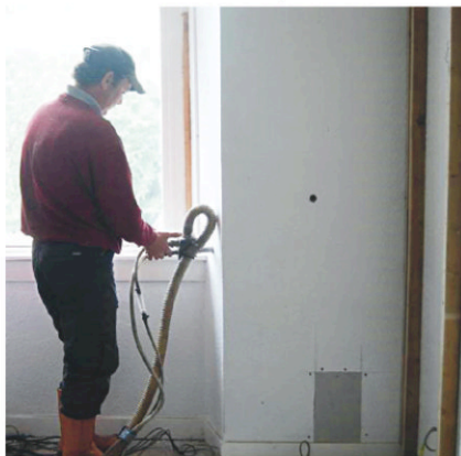
Figure 3 EPS beads were injected into the air spaces behind plasterboard in a Glasgow tenement building Copyright © Crown Copyright (Historic Scotland)
