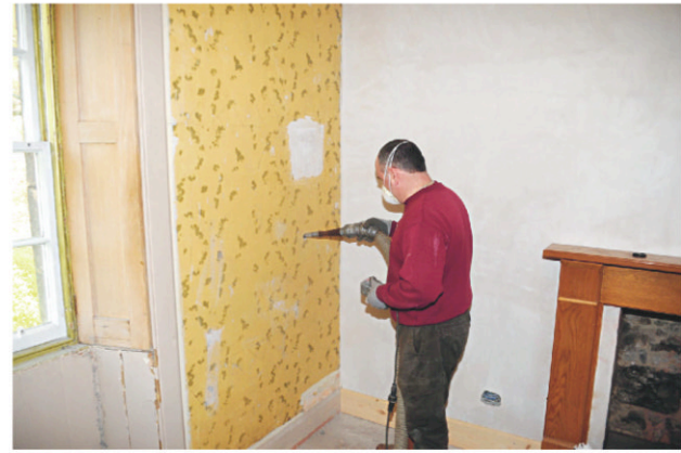
Figure 4 Insulating materials were injected into the air spaces behind plaster-on-laths finishes
