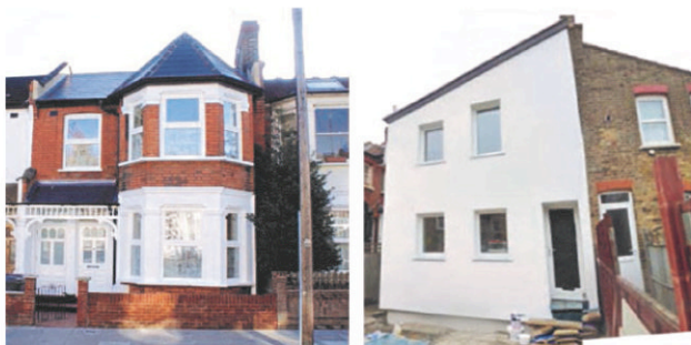
Figure 1 External wall insulation was only acceptable for use on the rear elevation of this mid-terrace house Copyright © Anne Thorne Architects.
