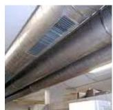
This ventilation systems are commonly used in crowded spaces where there are high internal thermal loads and there are high primary air ventilation rate requirements. All air system is composed by an Air Handling Unit (AHU) where the air is treated and then diffused into the rooms through ducts and air vents.
