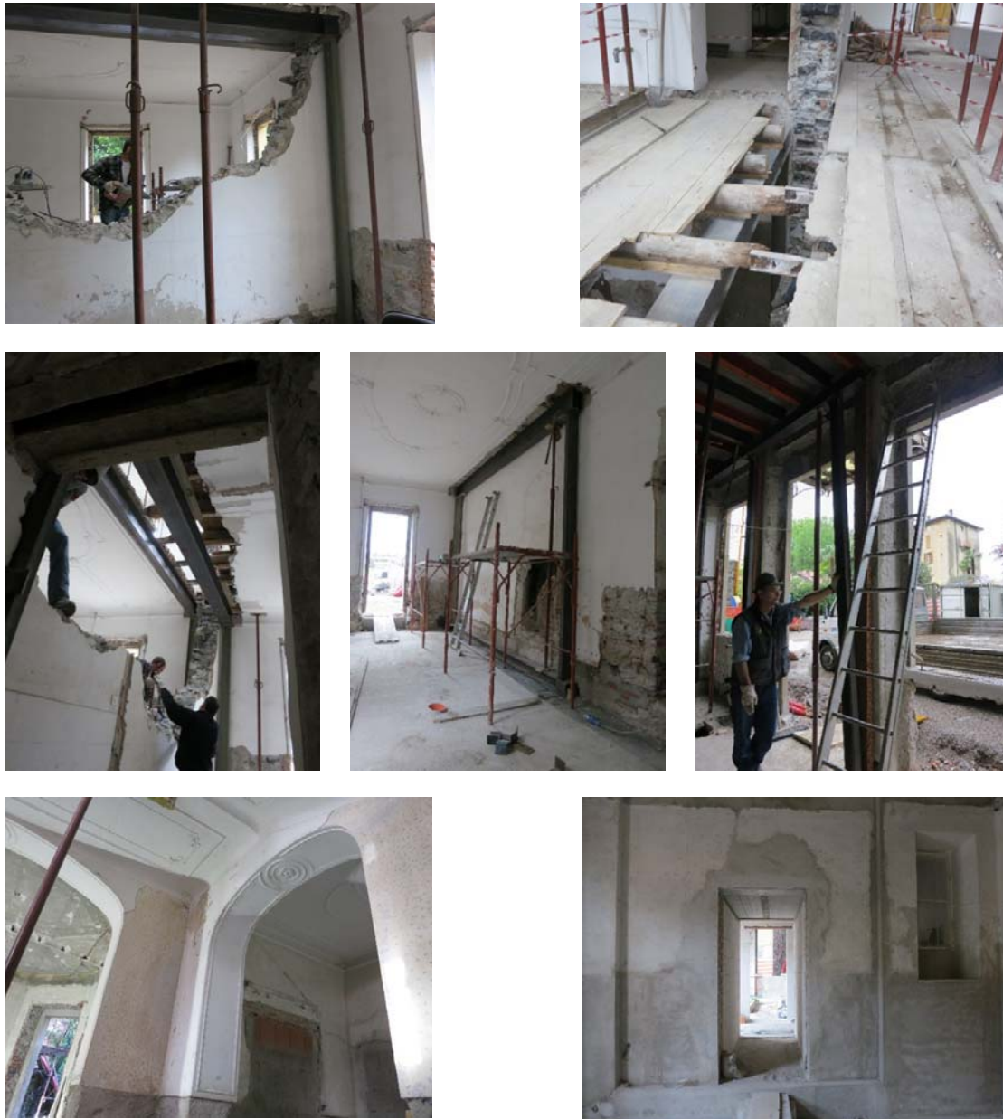
Figure 58-64: Work on the construction site
