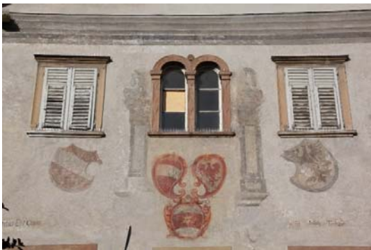
Figure 3: Fresco on south façade
