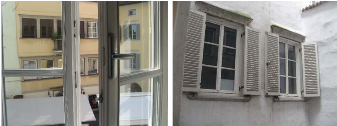
Figure 31-32: Windows used in the building
