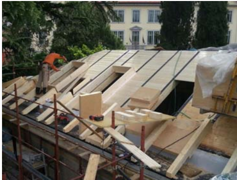
Figure 65-72: Work on the construction site
