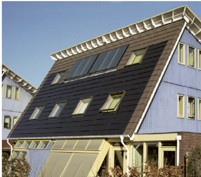
Figure 18: PV integration into a pitched roof (source: Avancis)
