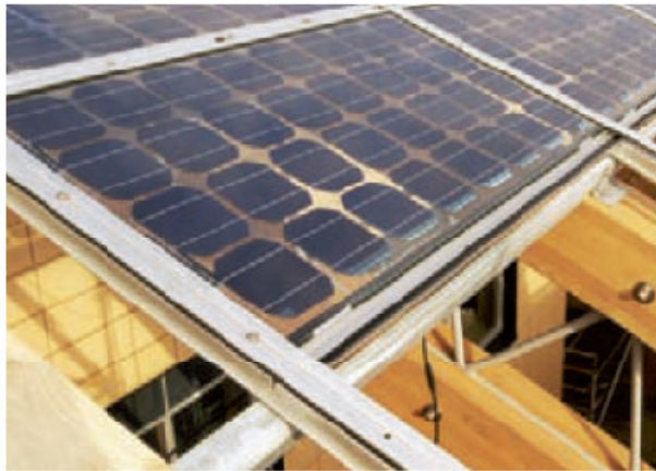
Figure 15: Monocrystalline PV in a semitransparent module (glass on the back). Photo courtesy: M.Art
