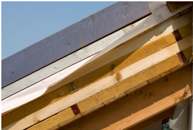
Figure 18 Use of cork boards for roof insulation
