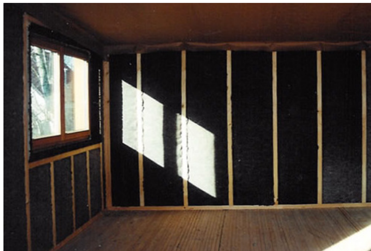
Figure 19 Internal insulation with sheep’s wool boards in between studs.
