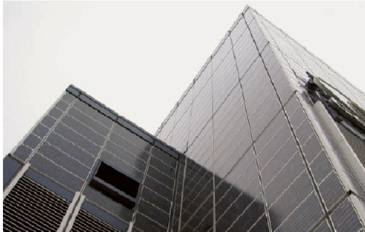
Figure 21: View onto the north west corner showing three types of cladding: cassettes of seven PV modules; narrower PV modules along the corners having identical appearance but electrically inactive; inexpensive coated steel dummy panels used around the vent.
