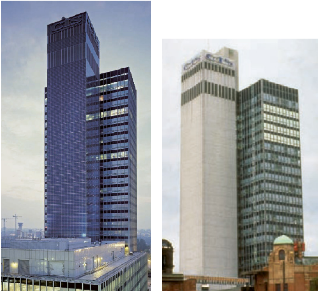
Figure 20: The Co-operative Insurance Tower after and before PV integration (Photo courtesy: Arup)
