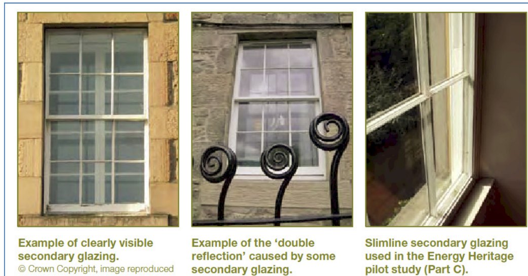
Figure 4 View from outside: visible secondary glazing (left), reflections and visual distortions (centre), secondary glazing without intermediate frames (right). 4
