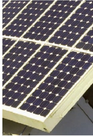
Figure 2: The G8 “solar showcase” BIPV pavilion built in 1998. This close-up shows the outline of monocrystalline cells within the modules. Photo: Christian Richters.
