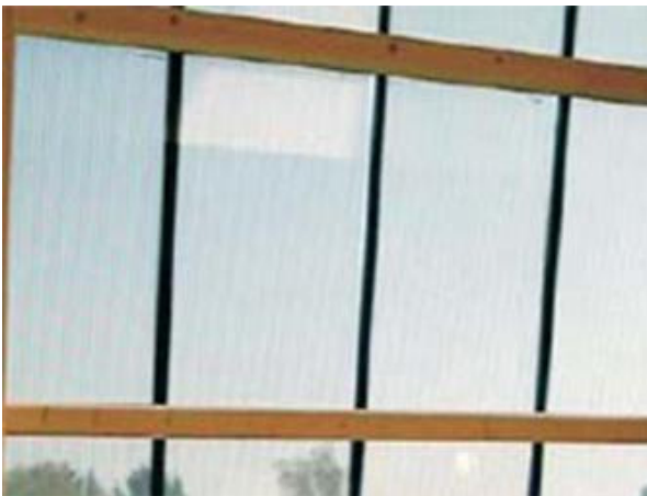
Figure 13: Roof application of Unisolar ASi thin film modules (source: Onyx Solar)
