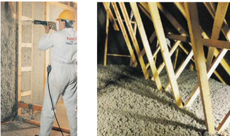
Figure 17 Cellulose flakes spray application (left) and roof sprayed insulation (right).
