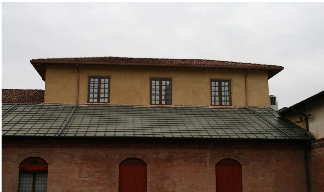
Fig. 11.9 Coat of Arms room outside windows detail
