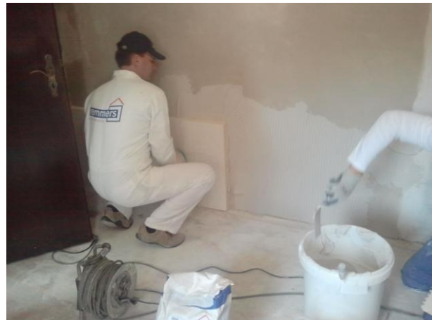
Applying of interior insulation
