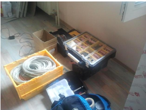
Preparation of monitoring installation
