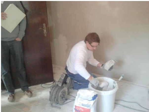
Applying of interior insulation
