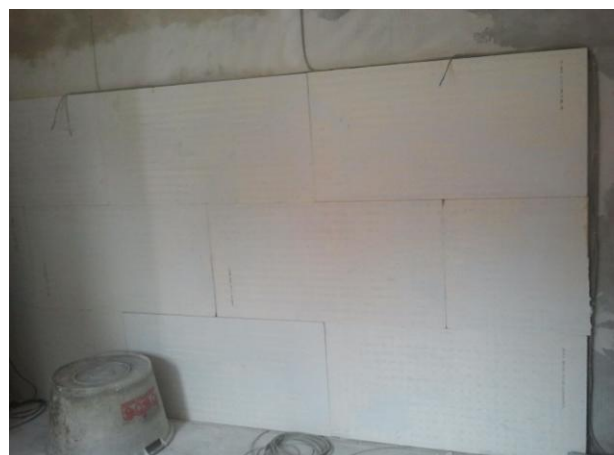
Complete the wall interior insulation with installation of different sensors
