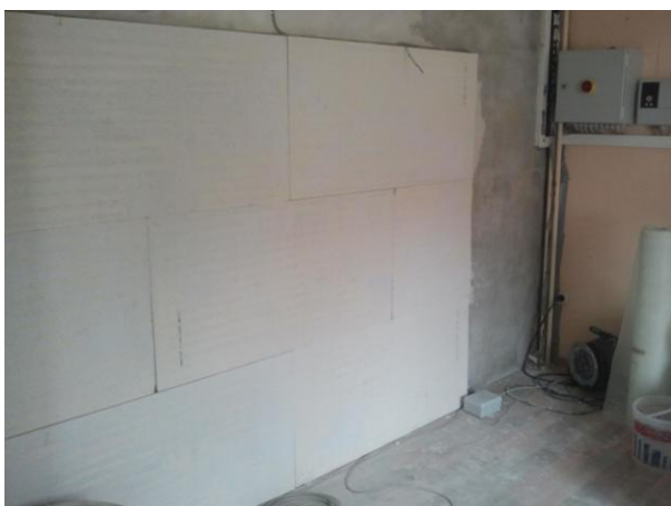
Complete Applying the wall interior insulation with installation different sensors
