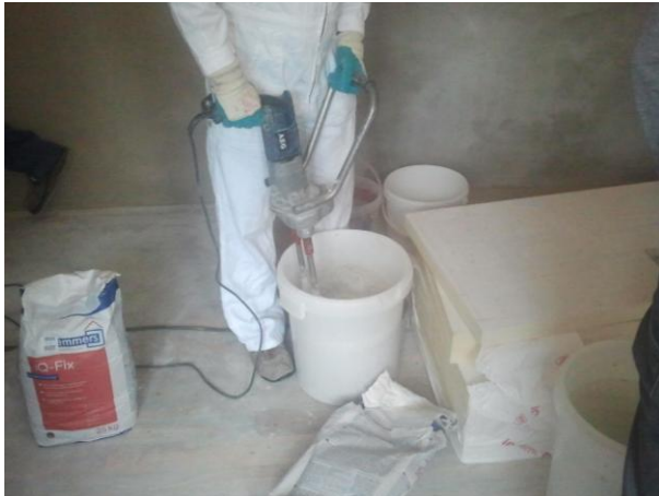
Applying of interior insulation
