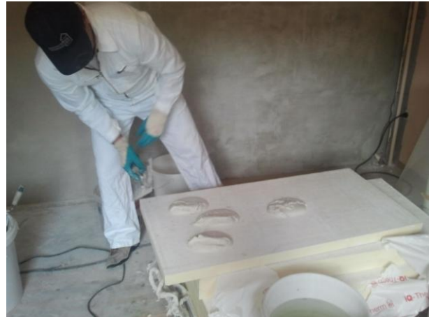
Applying of interior insulation
