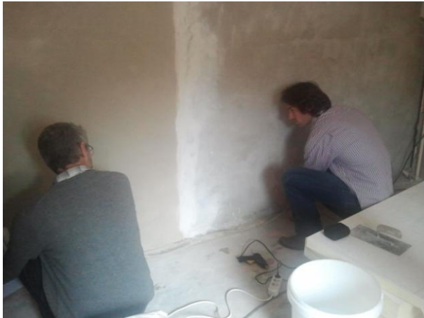
Installation of Sensors
