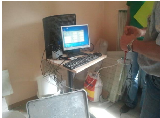
Complete the installation of Monitoring system
