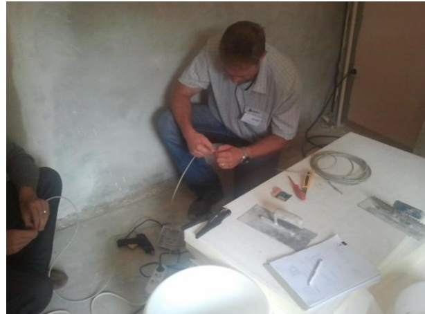
Insulation of Sensors
