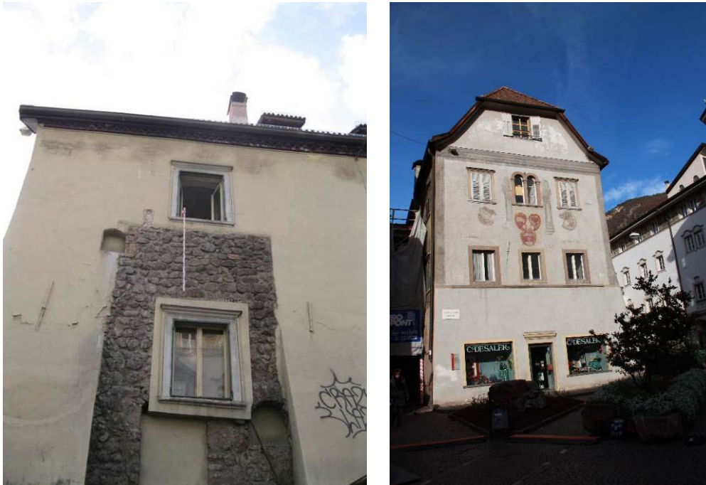
Figure 2.1: East and south façade of the building
