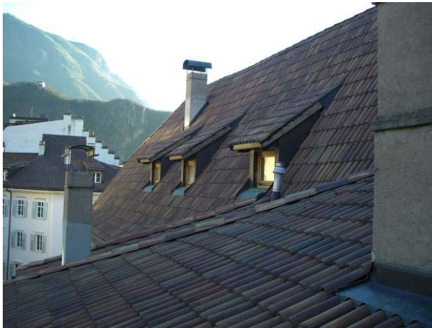
Figure 2.4: Roof dormers of the Weigh House
