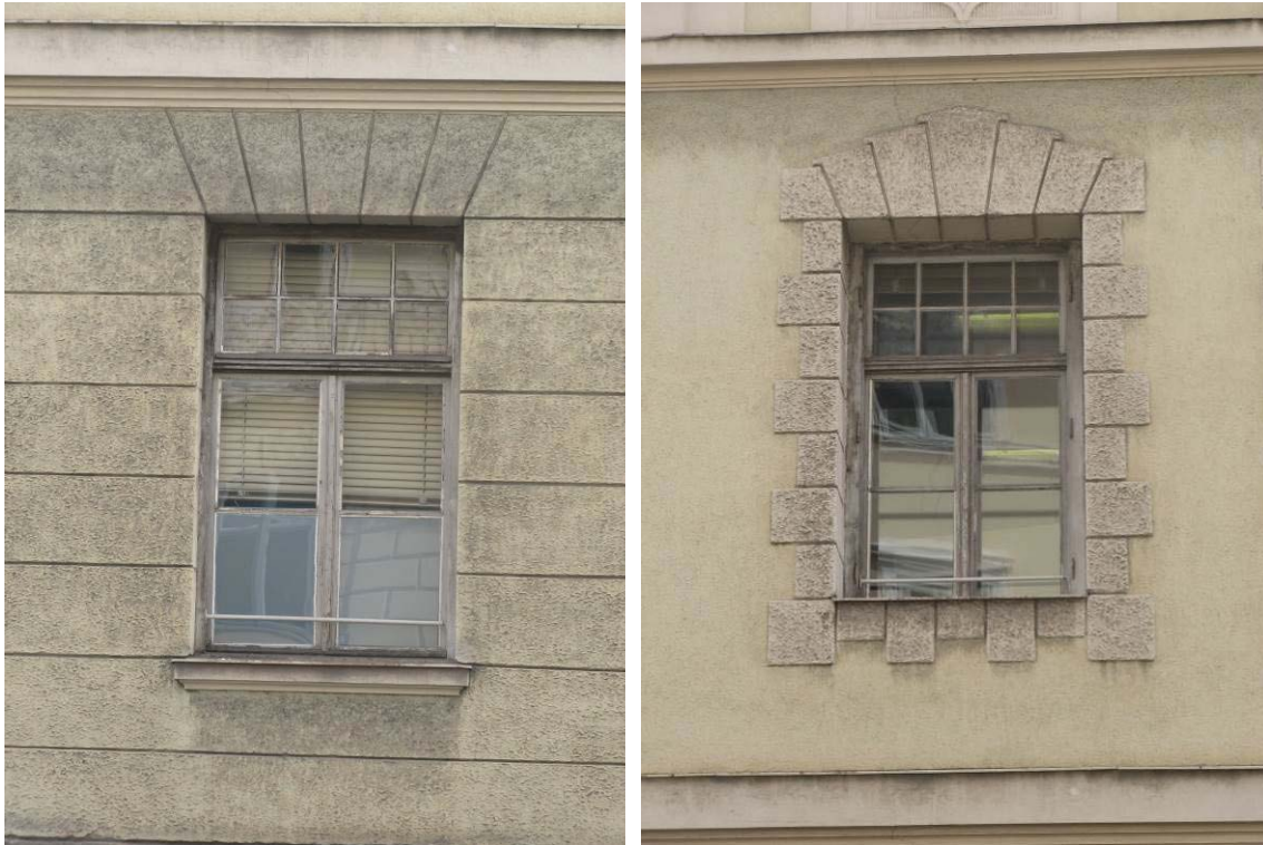
Figure 2.12: Box-type window of the “Aufschnaiter Middle School” in Bolzano
