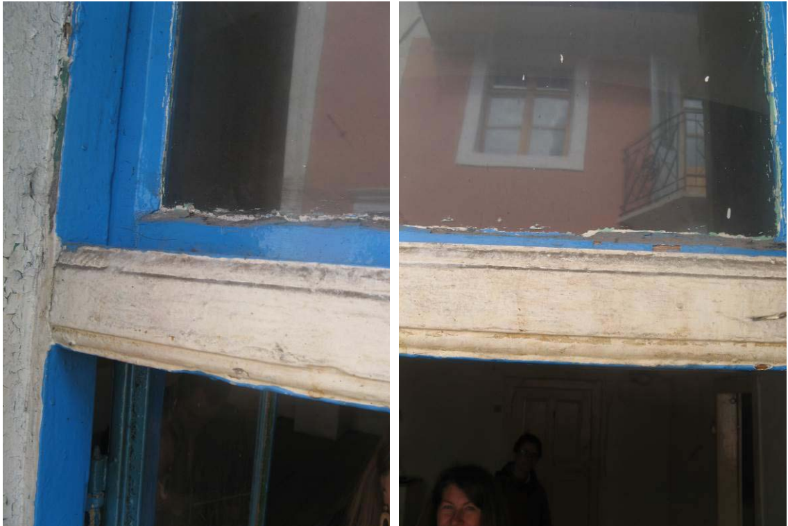
Figure 2.9: Shape of the impost at the bay window on second floor
