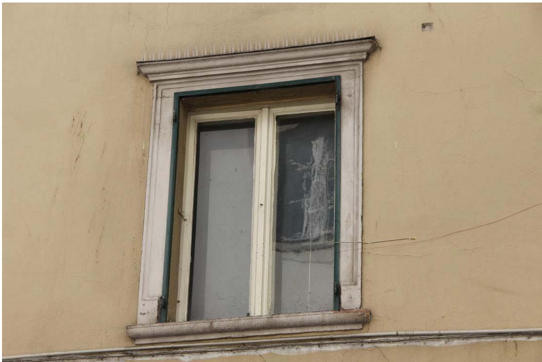
Figure 2.5: Existing window from the 50 th /60 th of the last century from inside and outside
