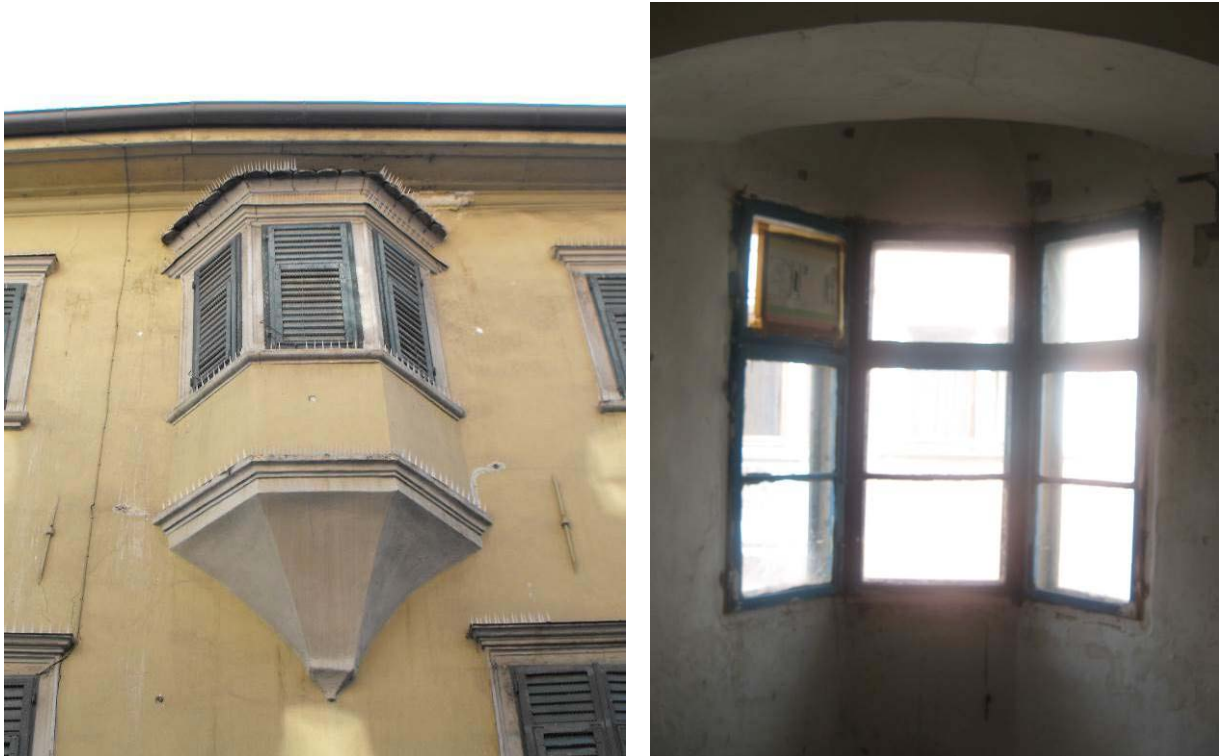
Figure 2.10: Bay window on second floor (from outside and from inside)
