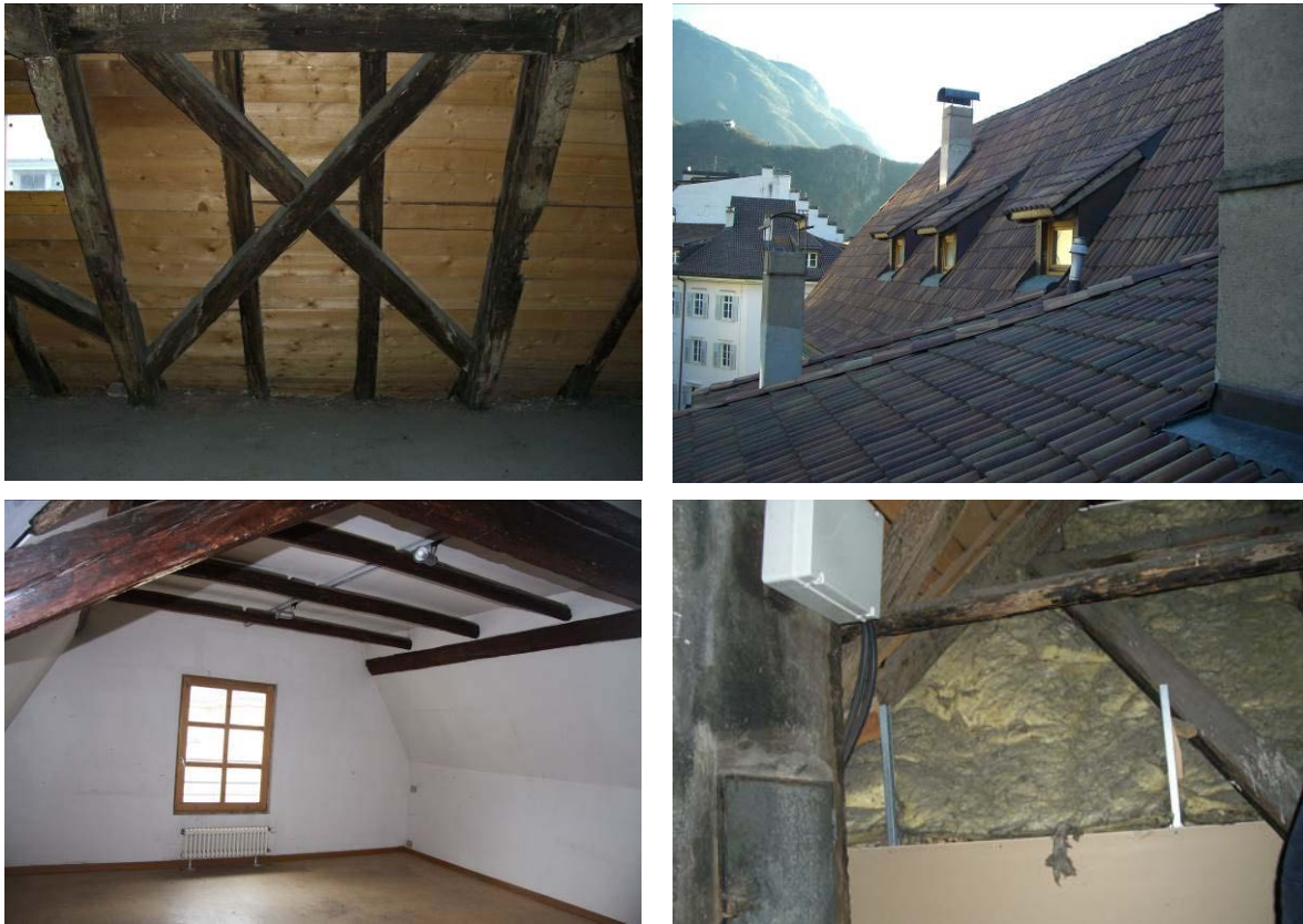
Figure 2.2: Roof of the building from outside and inside, isolated and non-isolated part
