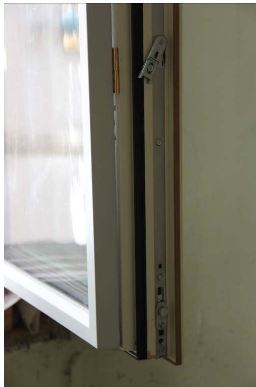
Figure 2.6: First high energy efficient window prototype installed in the Weigh House Comment by Dr. Kofler Engl (Director of the Heritage Office of South Tyrol) regarding the first window prototype, developed in the framework of the research project 3Encult:
